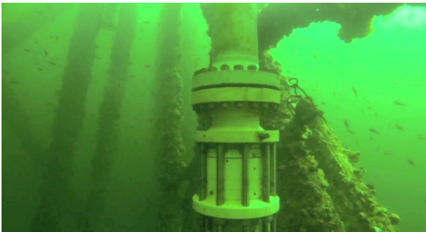
02 // MORGRIP® connector installed subsea onto vertical riser.
