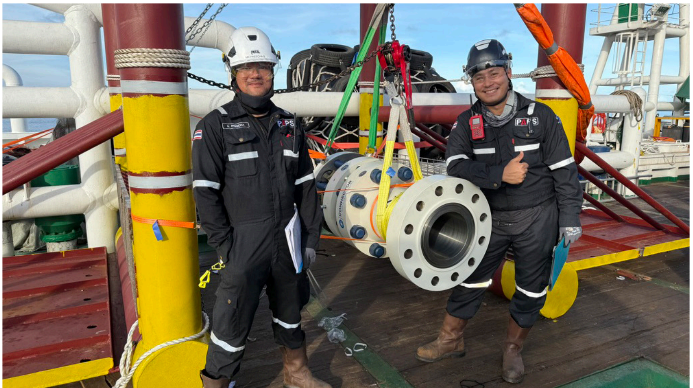
04 // CSS MORGRIP® Collet Connector offshore installation supported by PAPS technicians.
