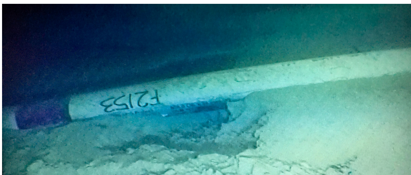
01 // ROV inspection of the planned clamp installation location.
