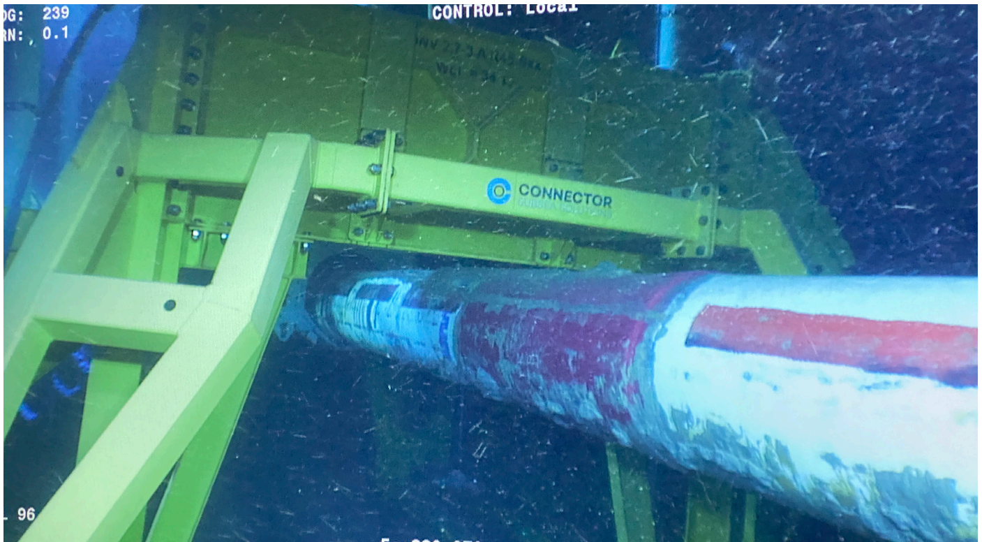
05 // Pipeline lifted to full height ready for sleeper installation
