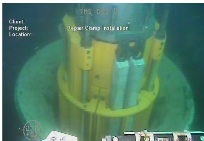
06 // CSS MORGRIP® Conductor Repair Clamp post repair ROV survey
