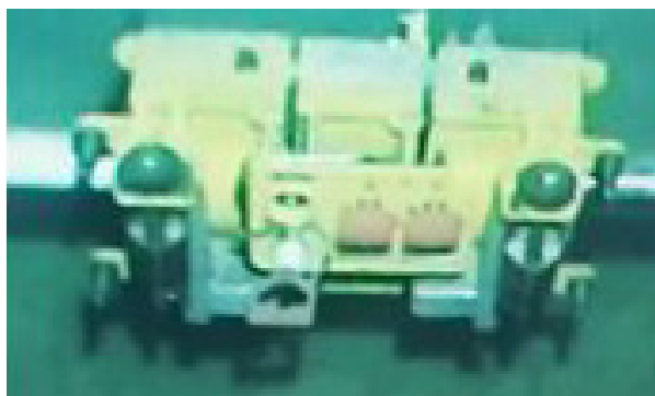
05 // CSS MORGRIP® 4" C-Bar Remote Clamp repair complete
