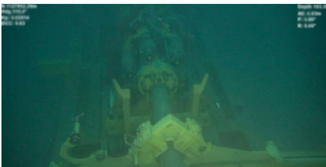
Connector activated on pipeline
